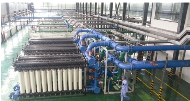
Fig. 6.48 Desalination device of independent microgrid system in Dafeng. Source China Jiangsu Website
